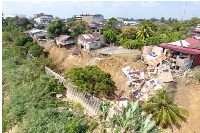
FIGURE 4. Failed Houses and Sheer Pile
